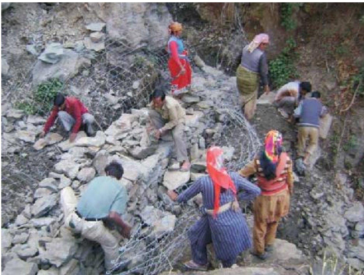
Villagers working on constructing a check dam as part of the catchment protection works at Village Ghogas, Jhaknidhar, Tehri, under WATSAN-II
