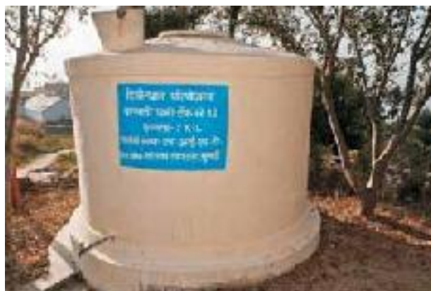
Rooftop rainwater tank- Village - Dhanaulti Laggagote, Tehri
