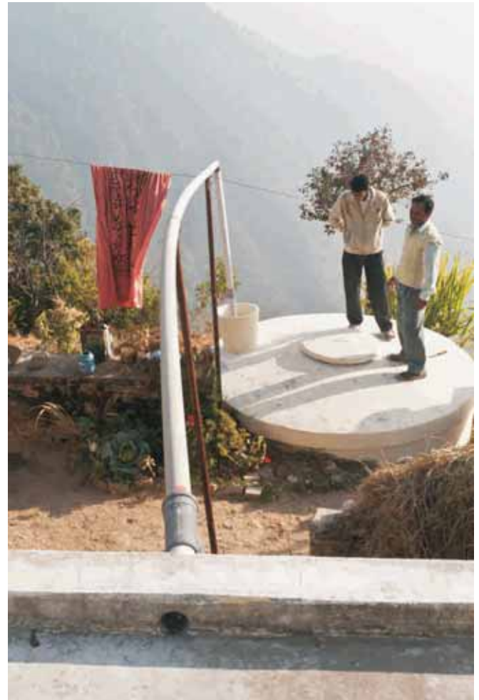
Roof Rain Harvesting Tank at village Churedhar Tehri
