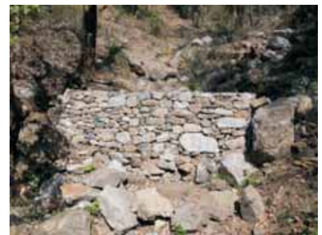
A check dam constructed by HERDS in the catchment of village Kushrella, Jaunpur. A total of 44 check dams were constructed in different areas.
