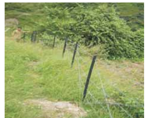
Fencing for protection of catchment area in village Bureck of Sirmaur district, Himachal Pradesh. A total of 436 rm fencing was done in 2012-13.
