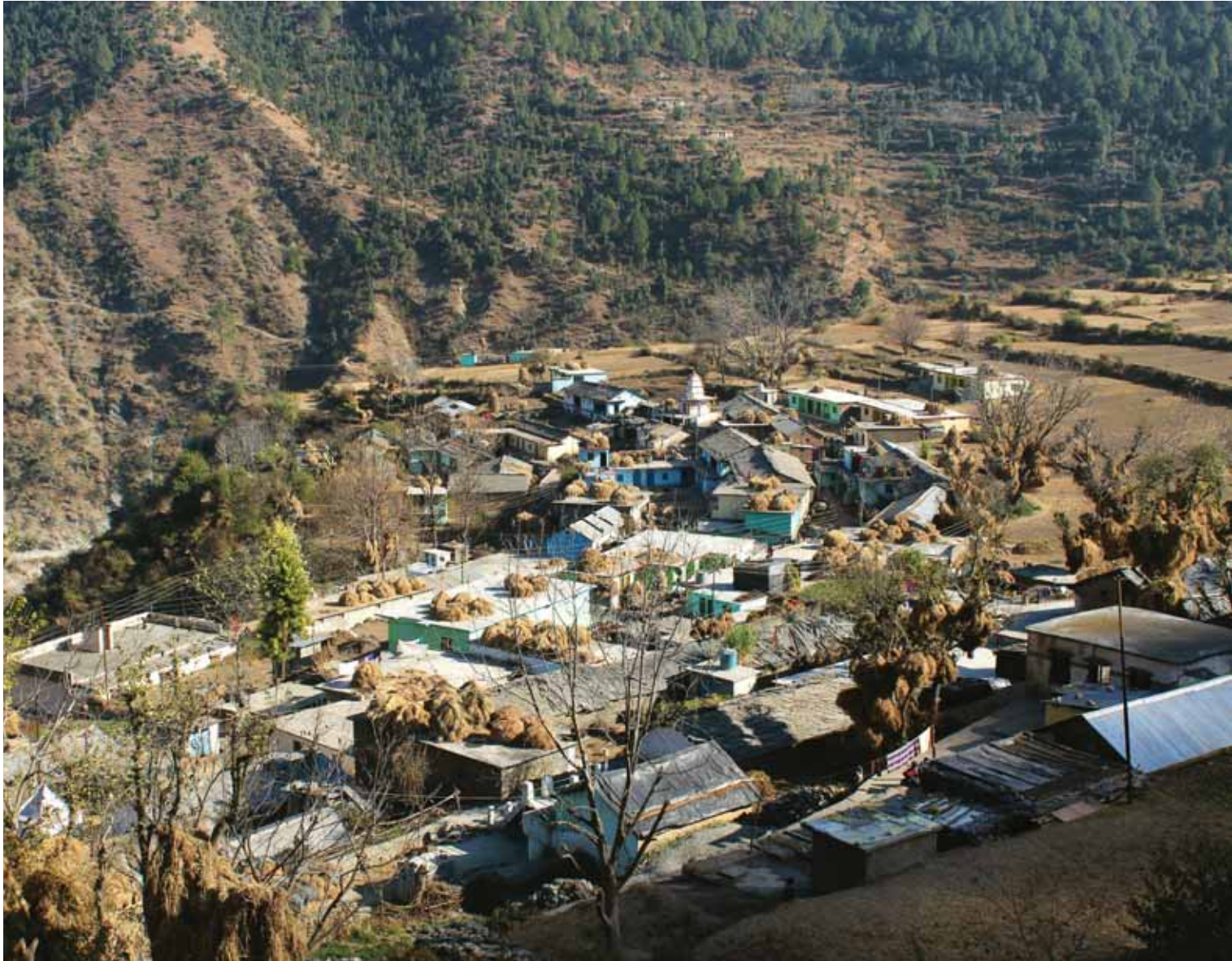
Almas village, Bhawan cluster, Tehri Garhwal
