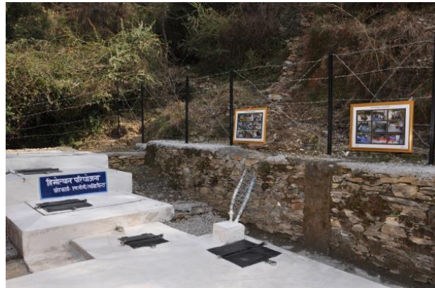
Spring water coming to the Sump and pumped to the Village through Submersible Solar pump
