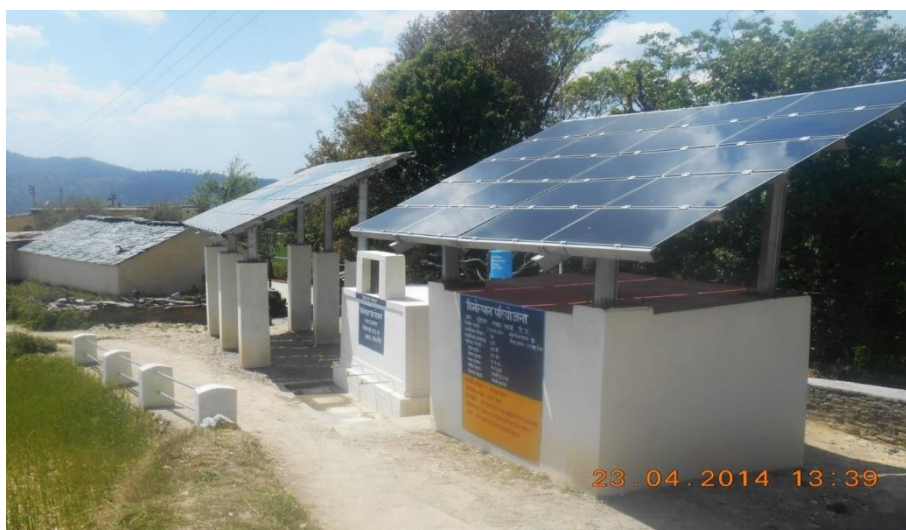
Two off line solar grid in the village producing 3,750 Wp to lift the water
